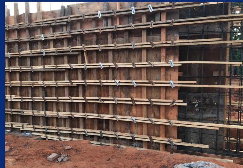
Concrete Wall Reinforcement and Forming at southeast corner of building
