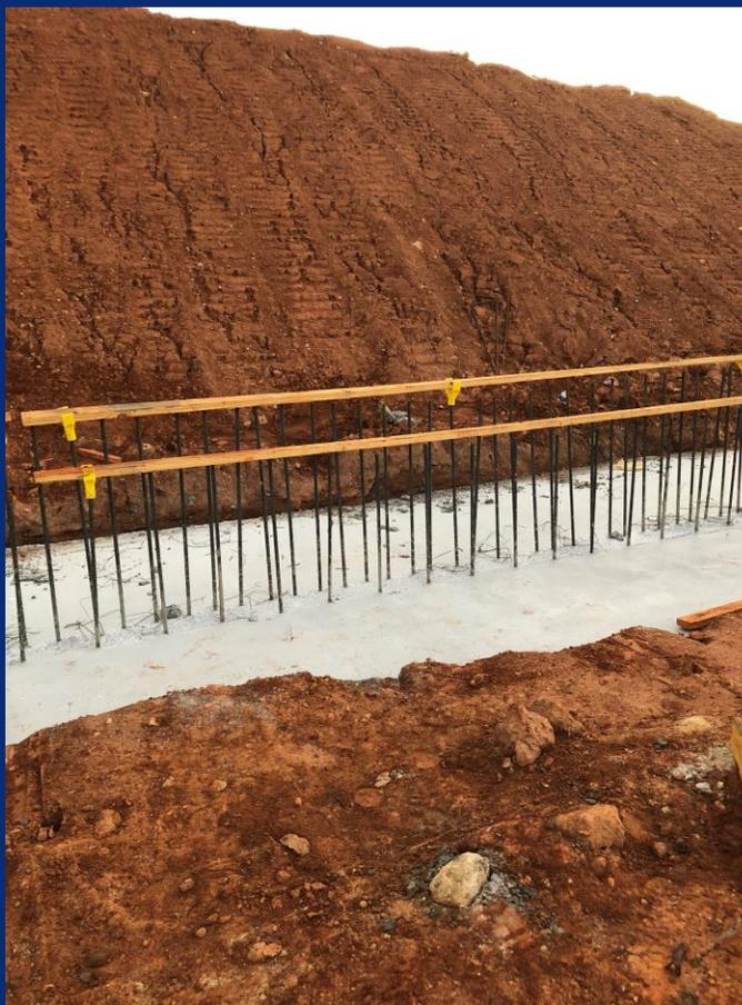
Foundation Concrete Poured at Building Retaining Wall
